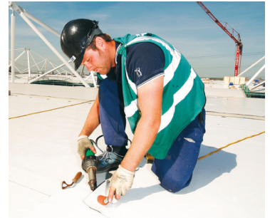
Forming a back weld
