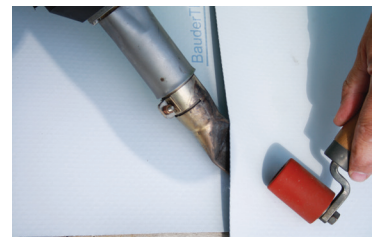
Forming a final weld
