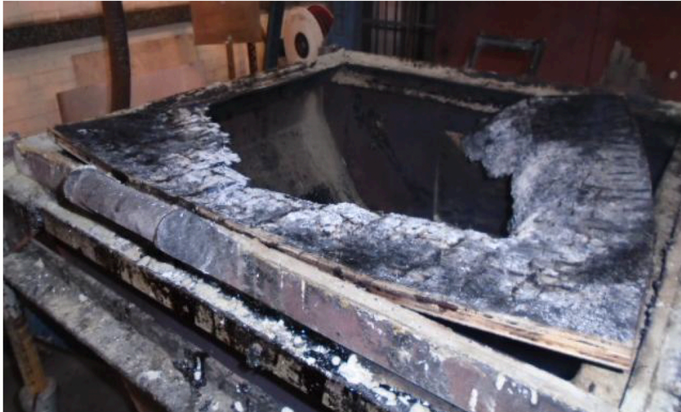
Figure 11- showing failure due to collapse of specimen 2 at 43 minutes.
